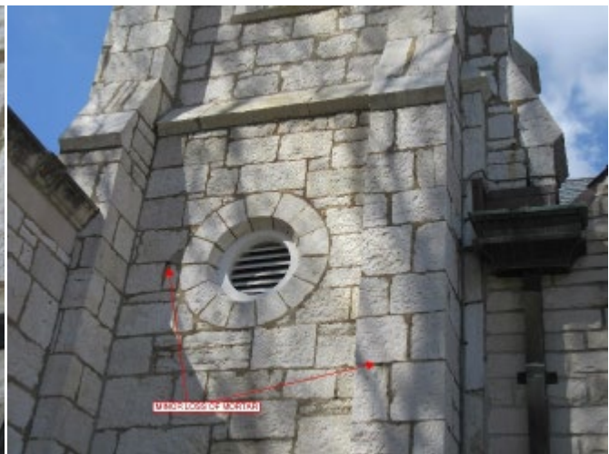
Minor cracking and mortar loss on exterior face of limestone walls
